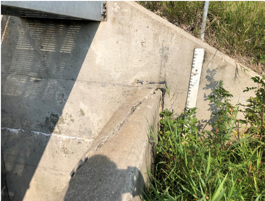
2020 WEIR WALL TO HEADWALL JOINT
