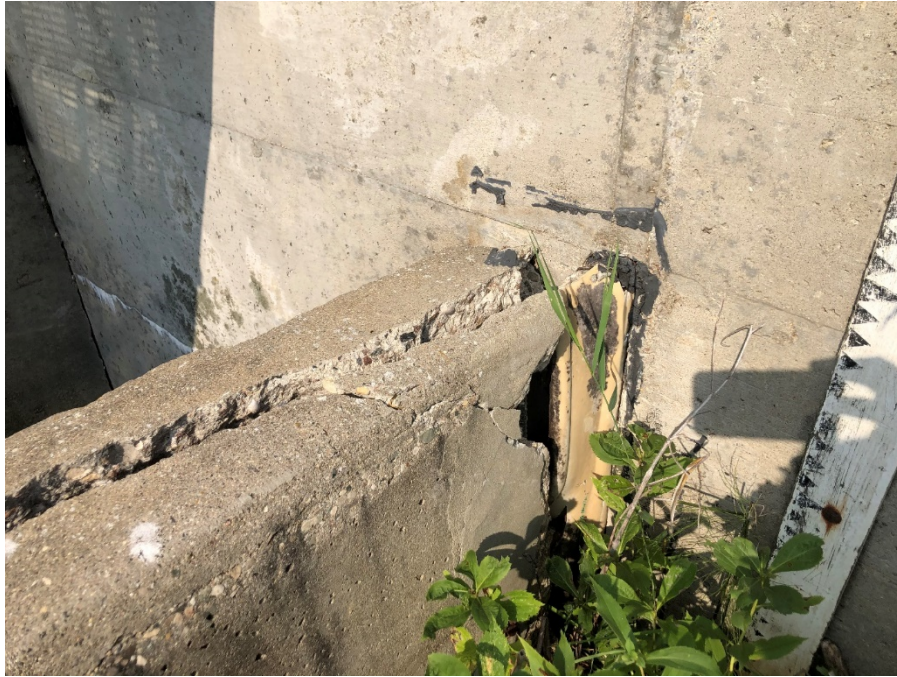
2020 WEIR WALL TO HEADWALL JOINT
