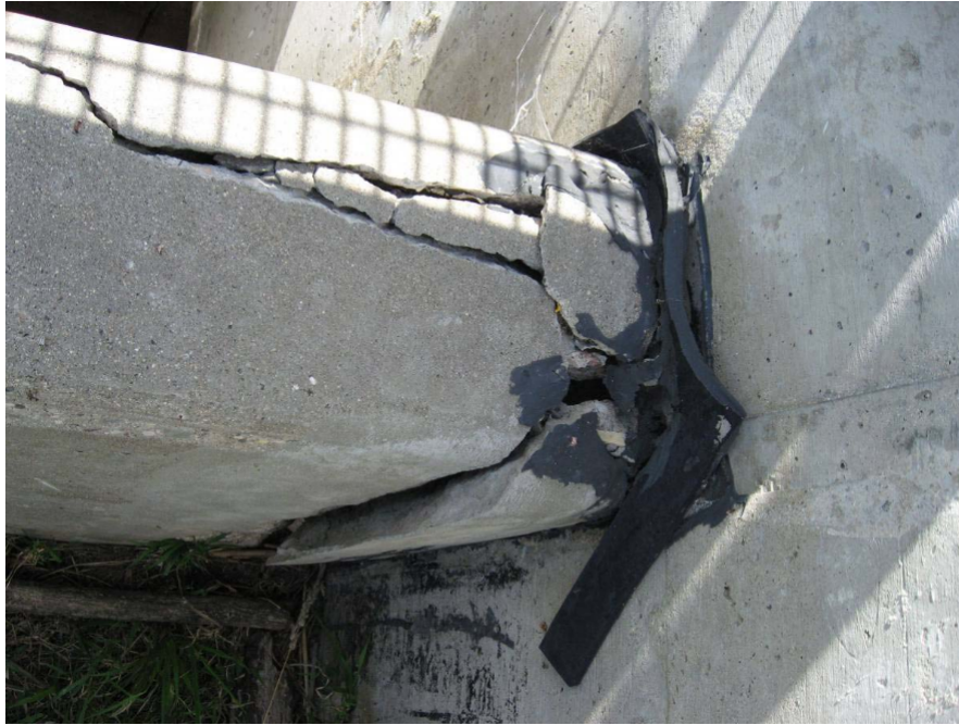
2007 WEIR WALL TO HEADWALL JOINT
